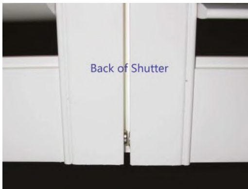
(2) Magnet keeping panels together
